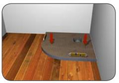
Place the Shower Tray into position and bed down onto the adhesive cement. Check that the shower tray is level in both directions using a suitable level.
