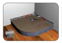
11. Where the shower area meets the wall apply a thin layer of tape sealer to the shower area and the adjoining wall approximately 60mm wide on both.
