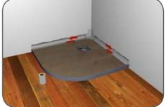
12. Place the strips of Waterproofing Tape previously cut in Step 7 along the edges of the shower area, folding half up the wall and half on the shower area as you go. Press firmly into the tape sealer and the tape should also overlap the Waterproofing Internal Corners. When you have finished you can remove the protective gloves and eye and breathing protection.
