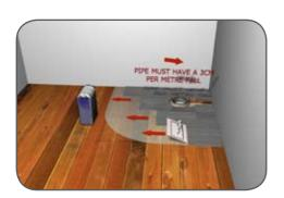
3. Note: Wear protective gloves, eye and breathing protection. Mix the board fixing adhesive according to the manufacturer's instructions to achieve a stiff consistency. Spread the board fixing adhesive onto the floor of the shower position and drag a 6mm notched adhesive trowel across the surface. The notched adhesive trowel will make a ribbed pattern which will leave just the right amount of adhesive on the floor.
