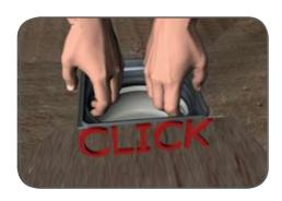
Put your finger through the drain hole in the Shower Tray. Push down on the Shower Tray and pull the Shower Drain upwards until it clicks into place into the drain hole in the Shower Tray.
