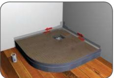
12. Place the strips of Waterproofing Tape previously cut in Step 7 along the edges of the shower area, folding half up the wall and half on the shower area as you go. Press firmly into the tape sealer and the tape should also overlap the Waterproofing Internal Corners. When you have finished you can remove the protective gloves and eye and breathing protection.
